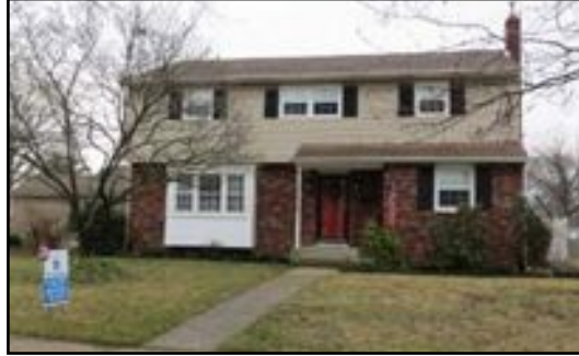
200 Madison Avenue Barrington/Gardens $274,900
